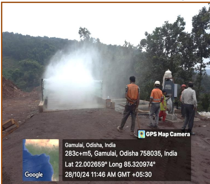
Photo-4 Wheel Wash Facility near exit gat
